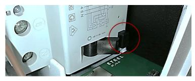
Figure 5: RCD test button
